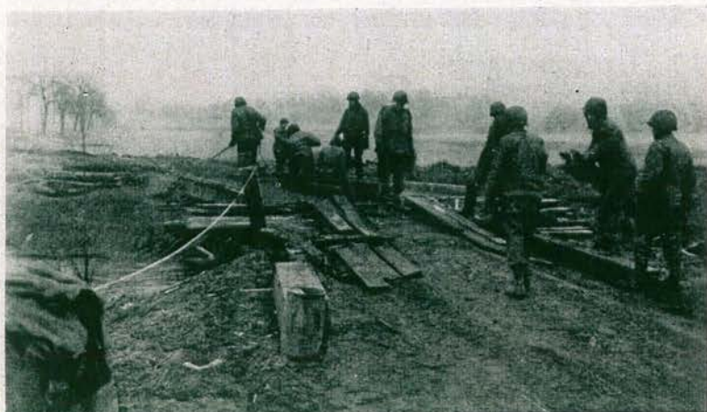
The first time we build timber trestle under treadway Hunspach, Alsace
