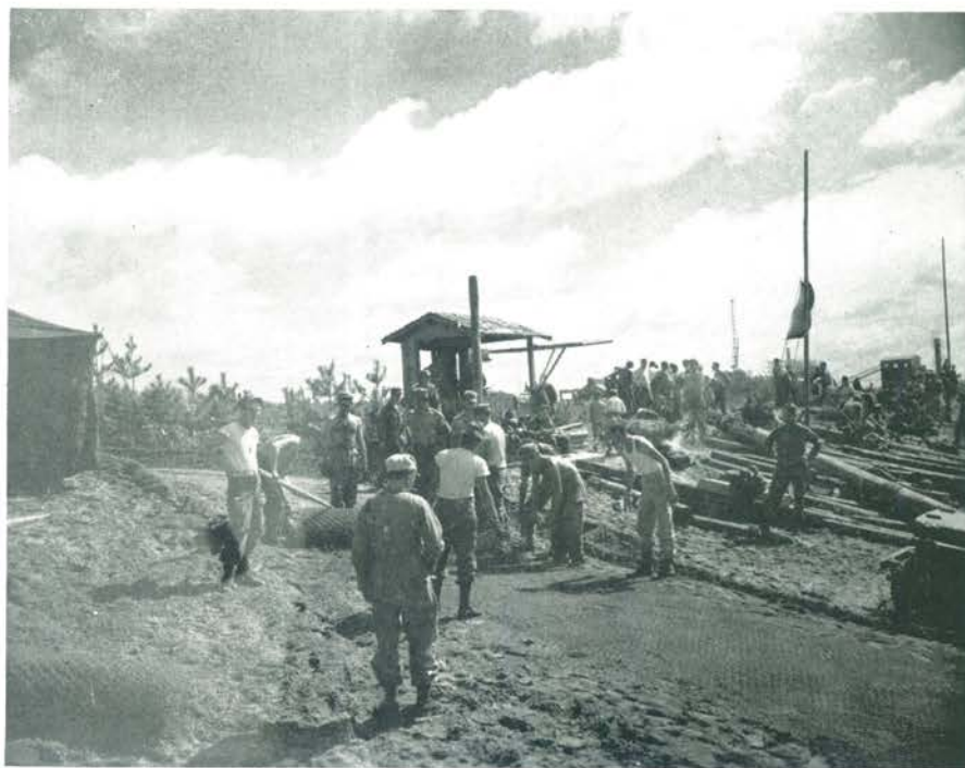
Temporary roadway of cyclone wire fencing is laid over the dunes to part of the dump area.
