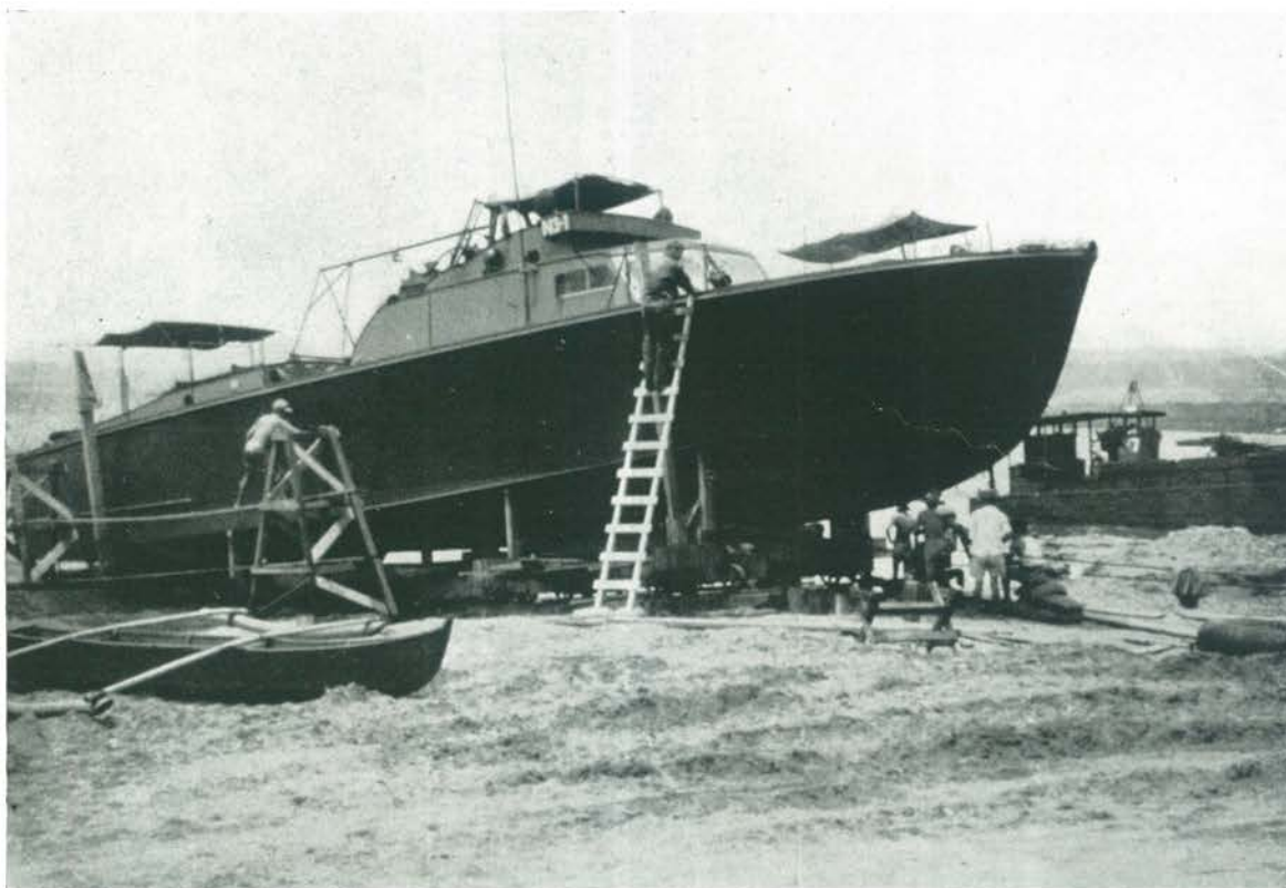
The marine railway at Bugo, built by A Company under the direction of T/3 Henry Moeller with the 50-ton 63-foot regimental command boat getting a new coat of paint.
