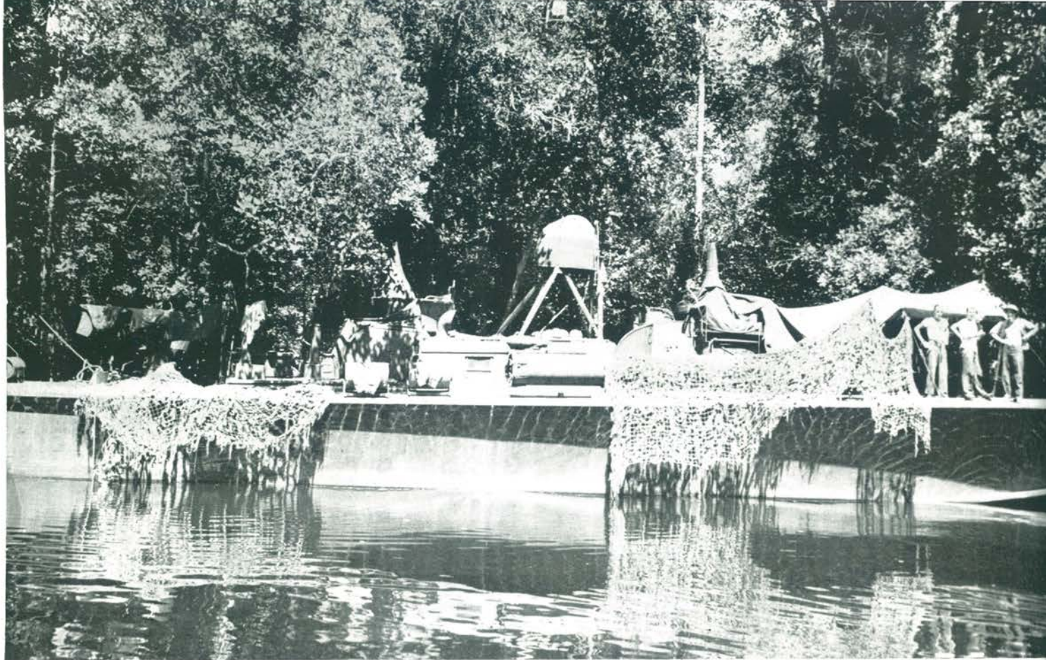
PT crews supplement the jungle concealment with camouflage nets at their base on the southern shore of Milne Bay.
