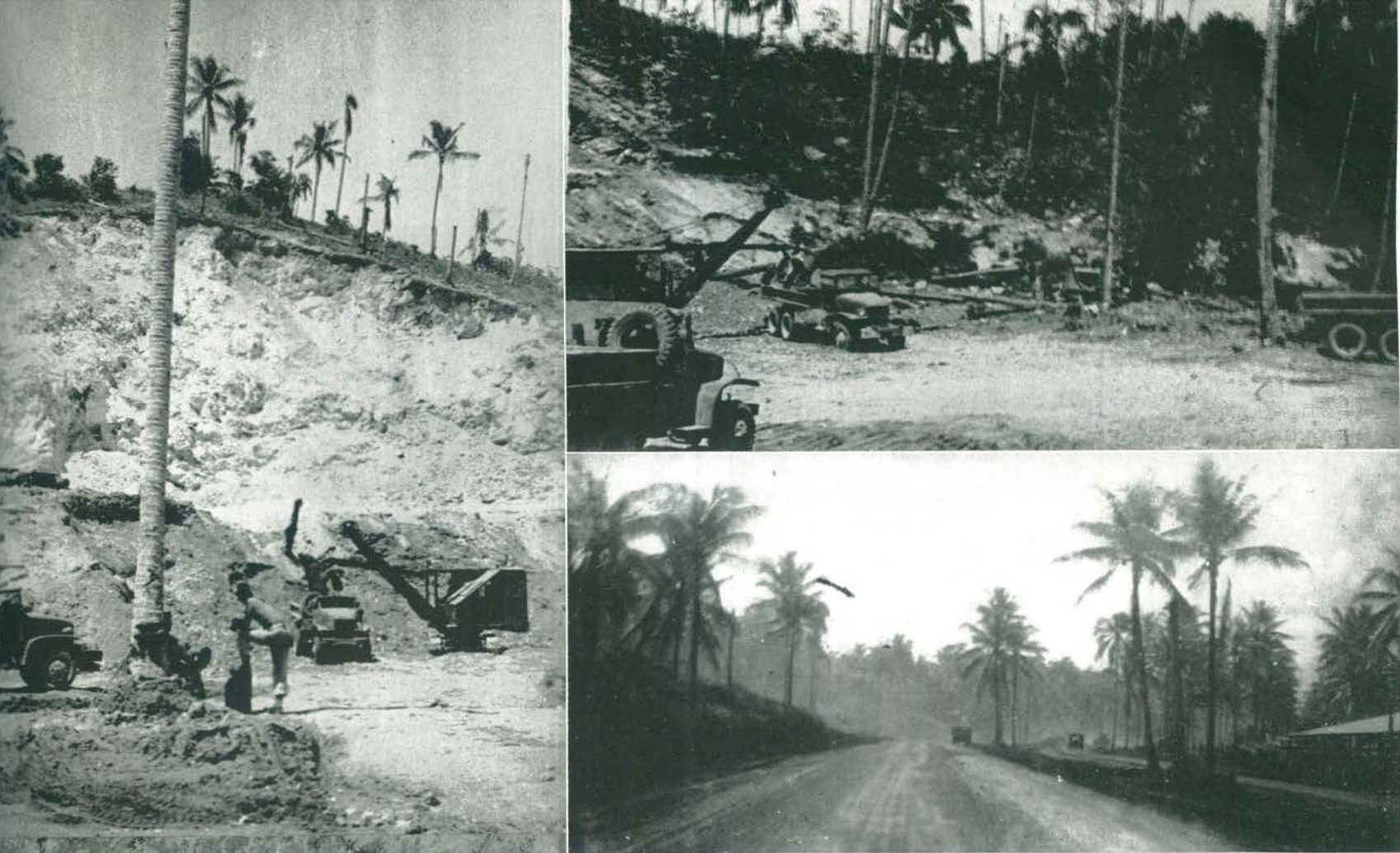
Left and upper right: Dipper stick filling dump trucks in borrow pit at Aitape.
