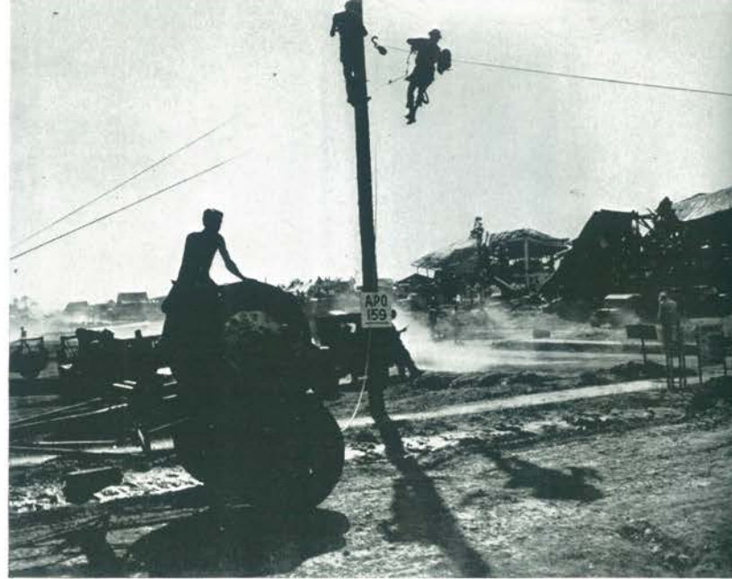
Stringing cable near Parang.
