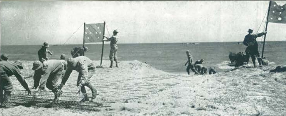
Top: Shore engineers erect beach markers and unroll strips of Somervell matting to provide a temporary road for vehicles soon to be landed.
