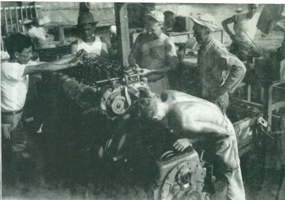
Tuning up a rebuilt Gray Marine Diesel in the 3d echelon shops of the 1461st.
