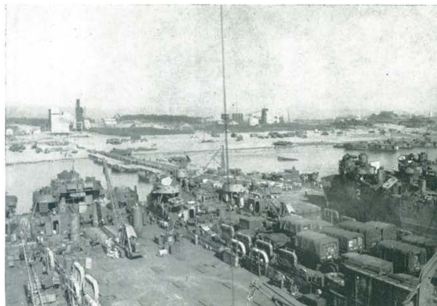
Jap jetty, extended by strings of ponton cubes, is used to discharge LSTs at first three at a time, later six at once.
