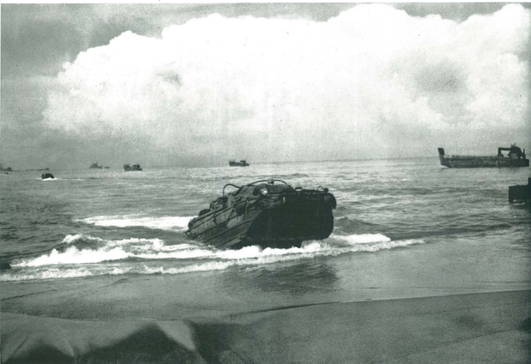
DUKWs and LCMs work side by side unloading ships over the beach at Cape Cretin.
