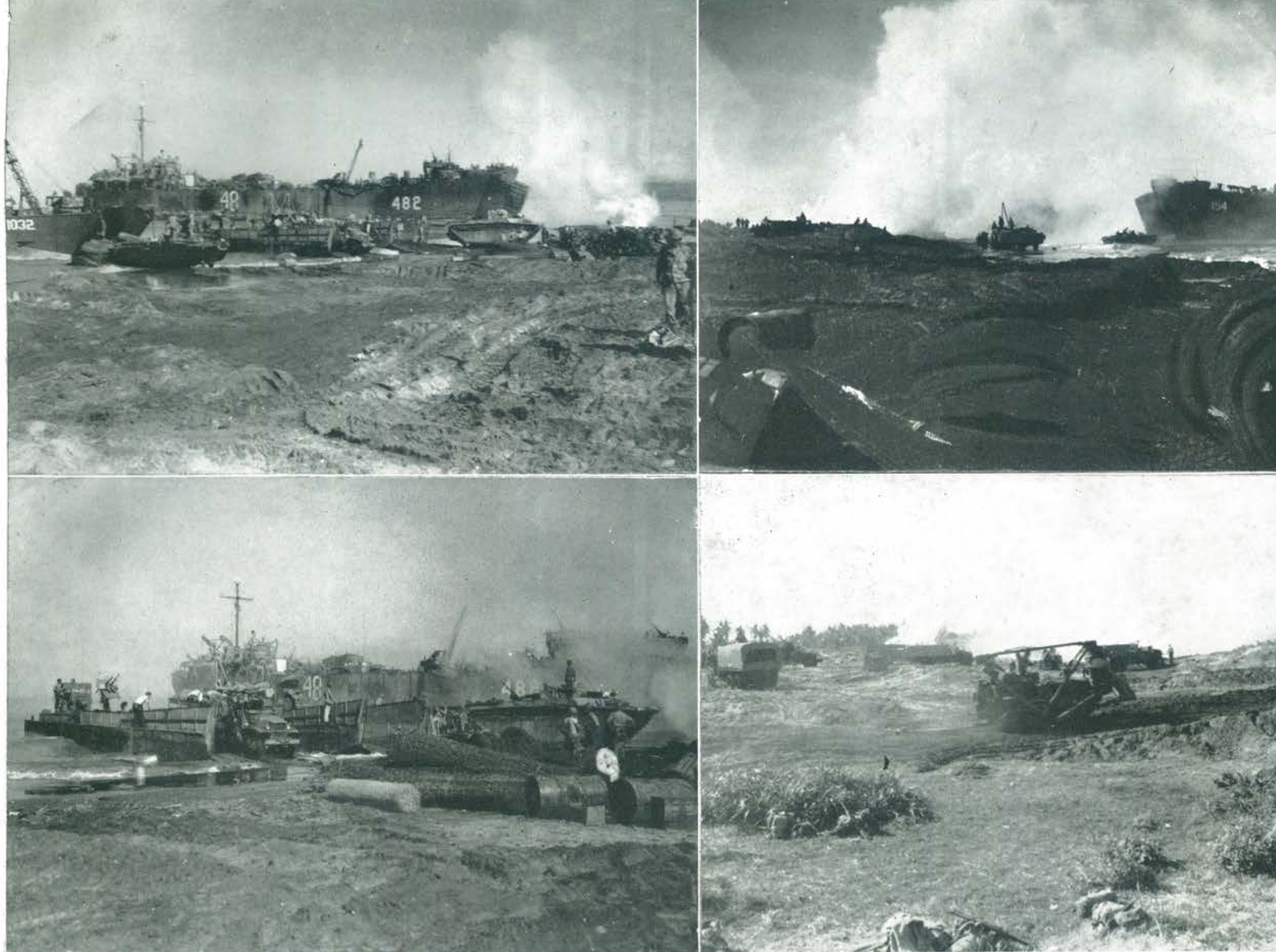
Beach White 2: Smoke pots conceal unloading operations from enemy observers in the hills and work continues despite intermittent shelling.
