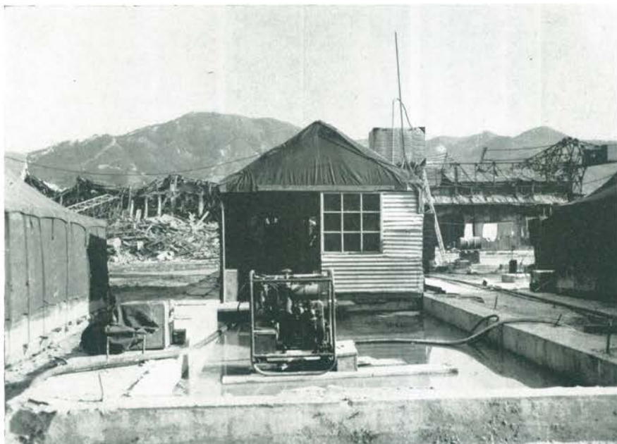
The Shore Battalion's Shower Room ( above ) with 2400 gallon hot water heating system constructed out of ponton cubes.
