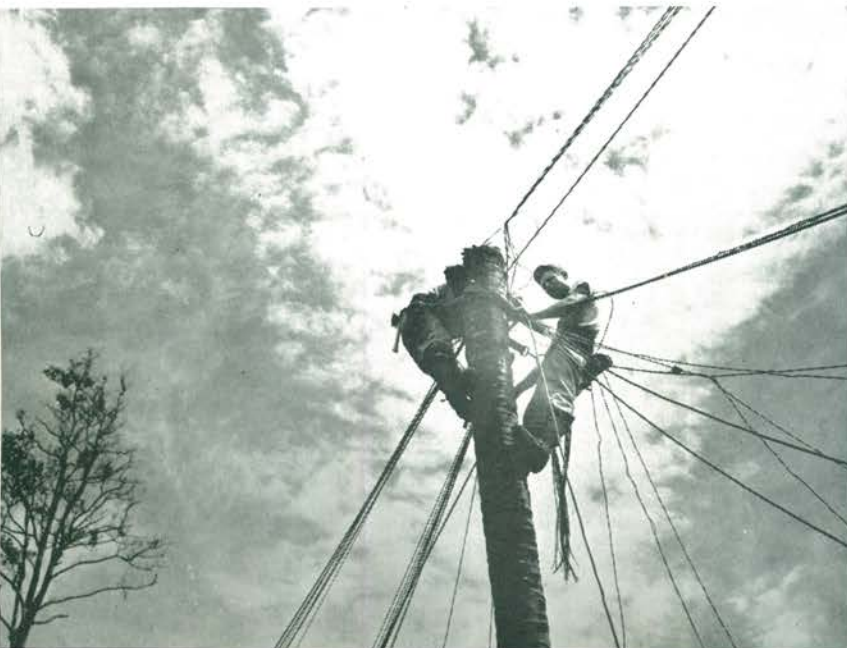
Keeping the wires identified on such a pole was no small job.
