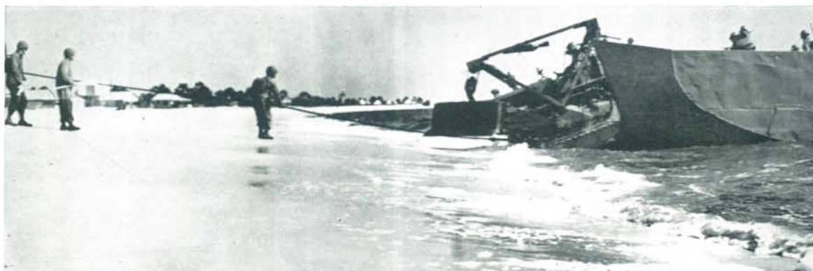
D-4 dozer slithers down the ramp of a Bureau-type LCM; note emergency tow line already fastened in case the dozer bogs down.
