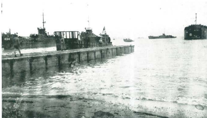
A section of ponton causeway is floated into position by an LCM.
