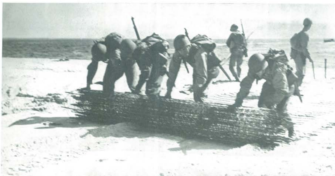
Shore engineers quickly lay beach matting over the soft sands of Red Beach.
