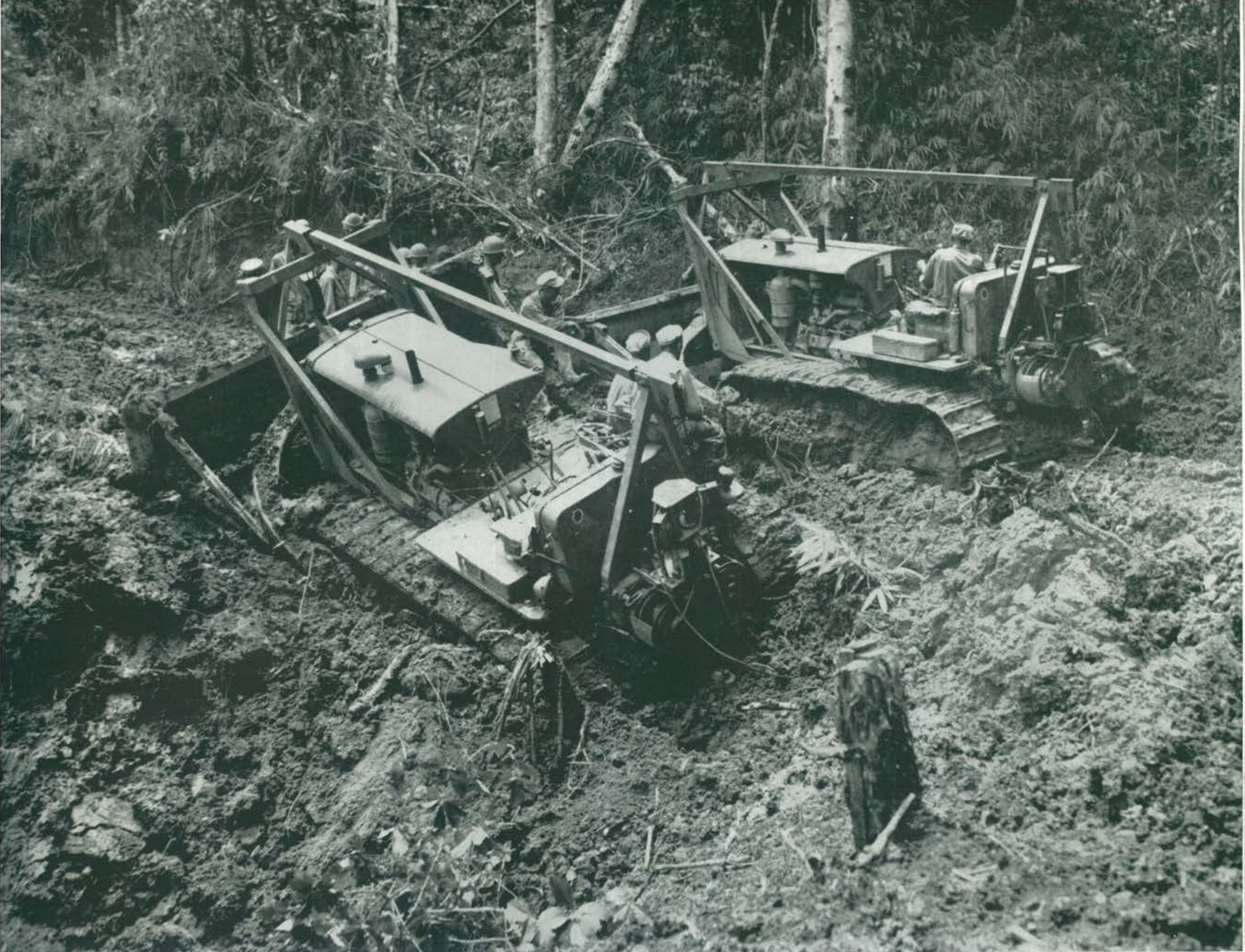
Mud was the curse of the early days at Saidor. Big dozers struggle to strip the jungle and make a river of goo into a road.
