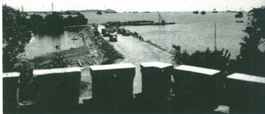
Jetty at Parang, as seen from the old Spanish Fort, after ponton cube extension enabled it to receive LSTs.
