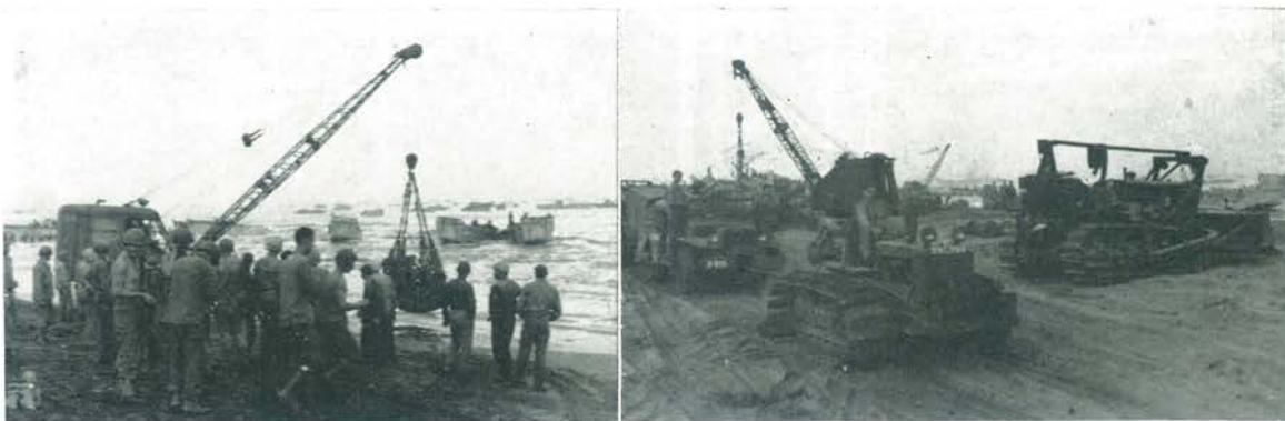
Beach White 3: Cranes expediting unloading and tractor towing disabled \frac{3}{4} -ton truck.
