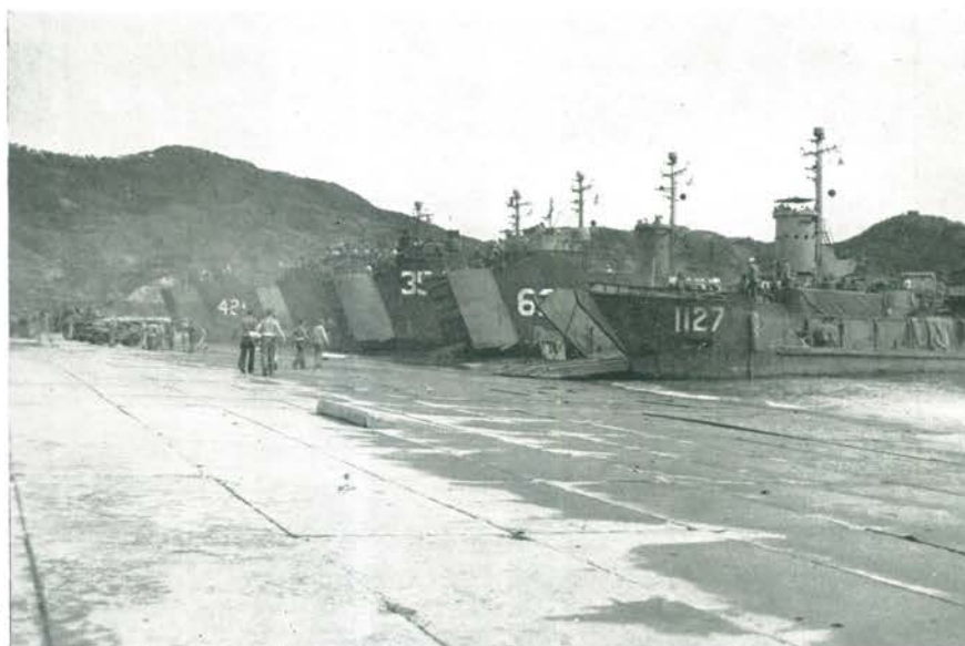
LCT and LSMs beached on the con- crete ramp of the Hiro Naval Air Station.
