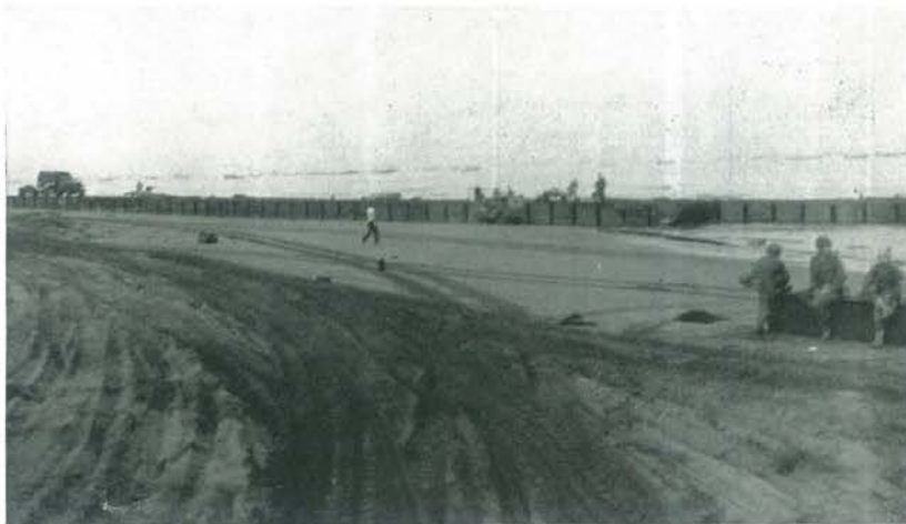
Ponton causeway broached between White 2 and White 3 is turned into bridge across mouth of slew.
