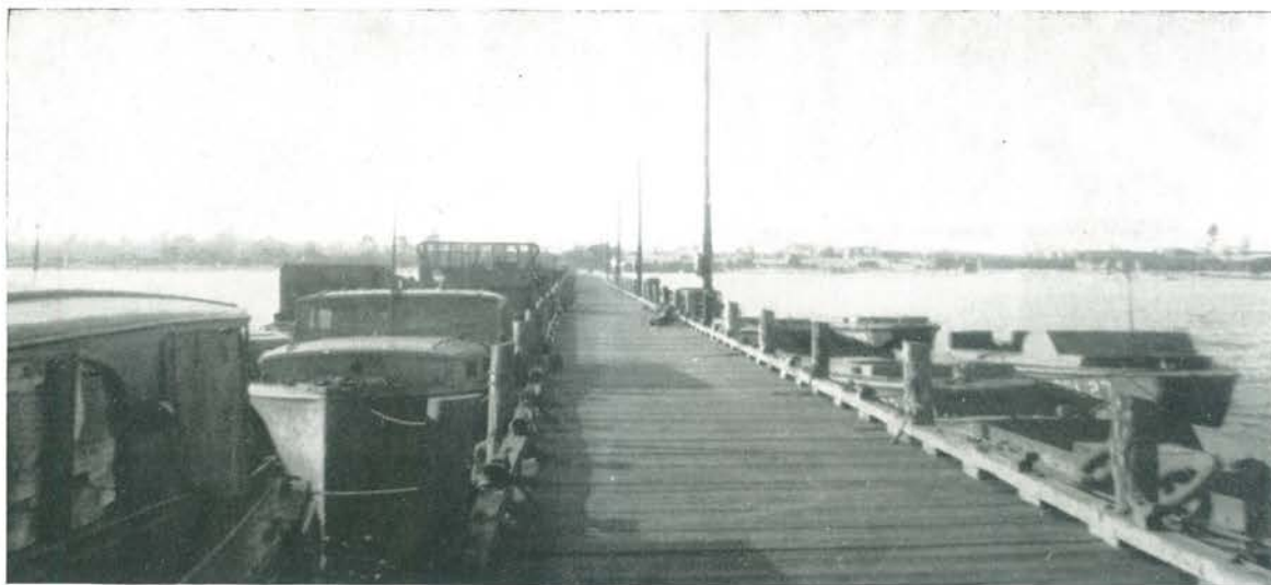
Pier 2, Carrabelle, looking shorewards; boats of Boat Battalion Headquarters Company in the foreground.
