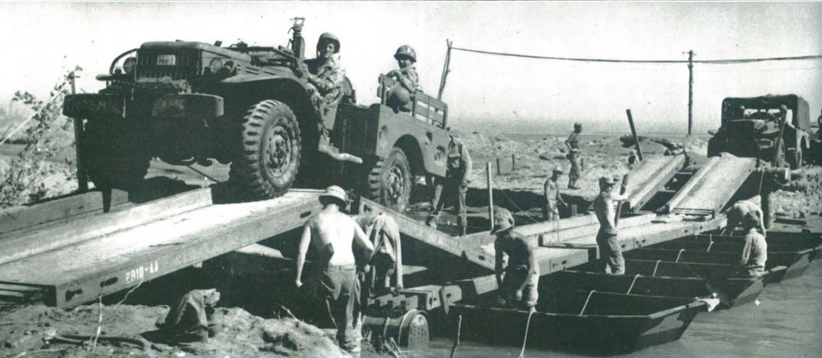
Top: A Shore Battalion DUKW rushes reinforcements from Aitape towards the Driniumor. Bottom: Treadway bridge across a slew near Anamö.
