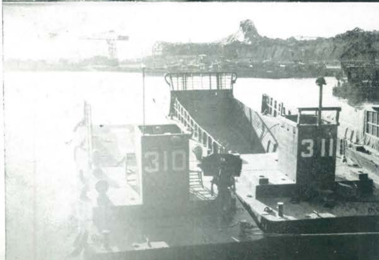
LCMs tied up outside the small boat basin. Note the ruins of the steel mill in the background and the large hammer-head crane used to lift out LCMs for repair.
