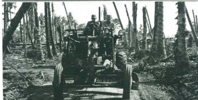
Front view of D-12 road grader.
