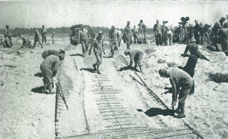
Bottom: The matting, of chicken wire stiffened with soft iron rods, is further strengthened with steel edge strips and staked down to prevent curling under the weight of the heavily loaded trucks.
