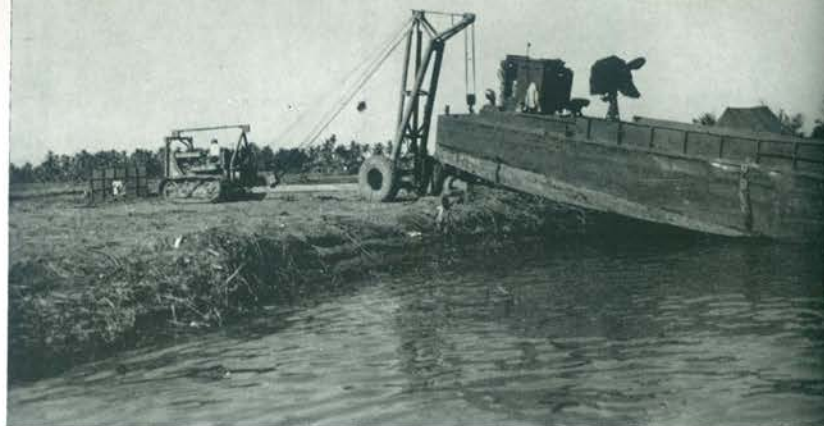
Hauling an LCM on the bank of the Bued River, Luzon.
