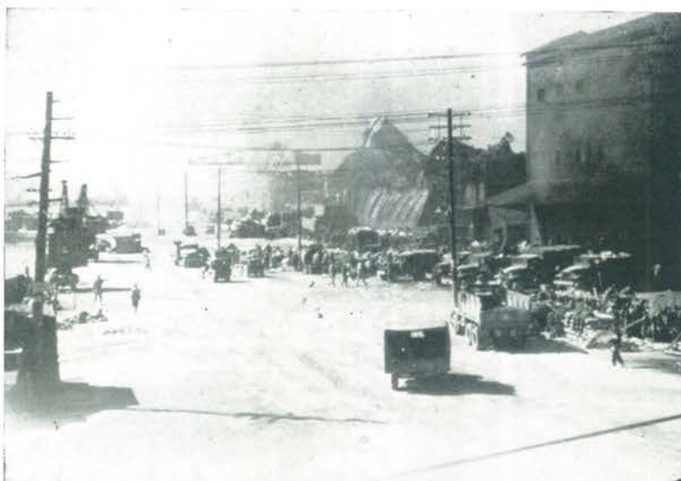
The parking area by the small boat basin in the Kure Mine Base.
