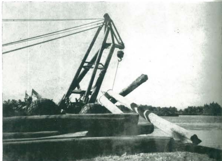
20-ton Letourneau tractor crane clearing logs.
