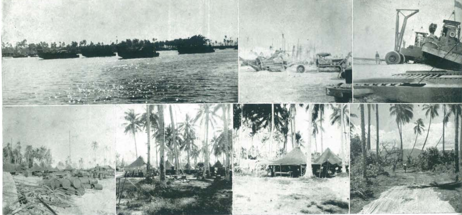
Scenes from Seleo Island: Left to right, top to bottom: The anchorage; carryall building beach over coral shelf; hauling an LCM on the artificial beach; vistas of C Company's bivouac; the island's only highway.
