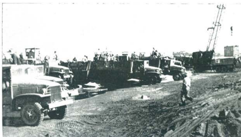
The LCM part of Beach White 2 in full operation with Filipino labor, February, 1945.
