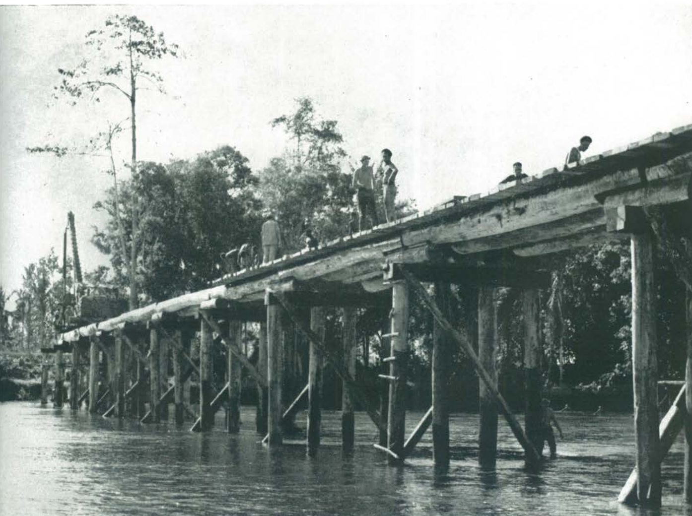
Typical trestle-bent bridge using a minimum of non-local materials.
