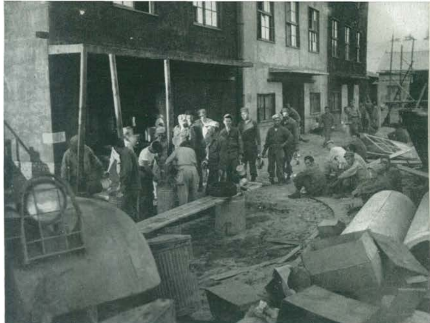
Regimental Headquarters Company's bivouac at Wakayama in the shell of a gutted steel mill.
