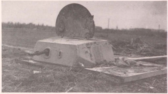
Armored pillbox in front of Niederzier. Camouflage was removed before taking the photo.
