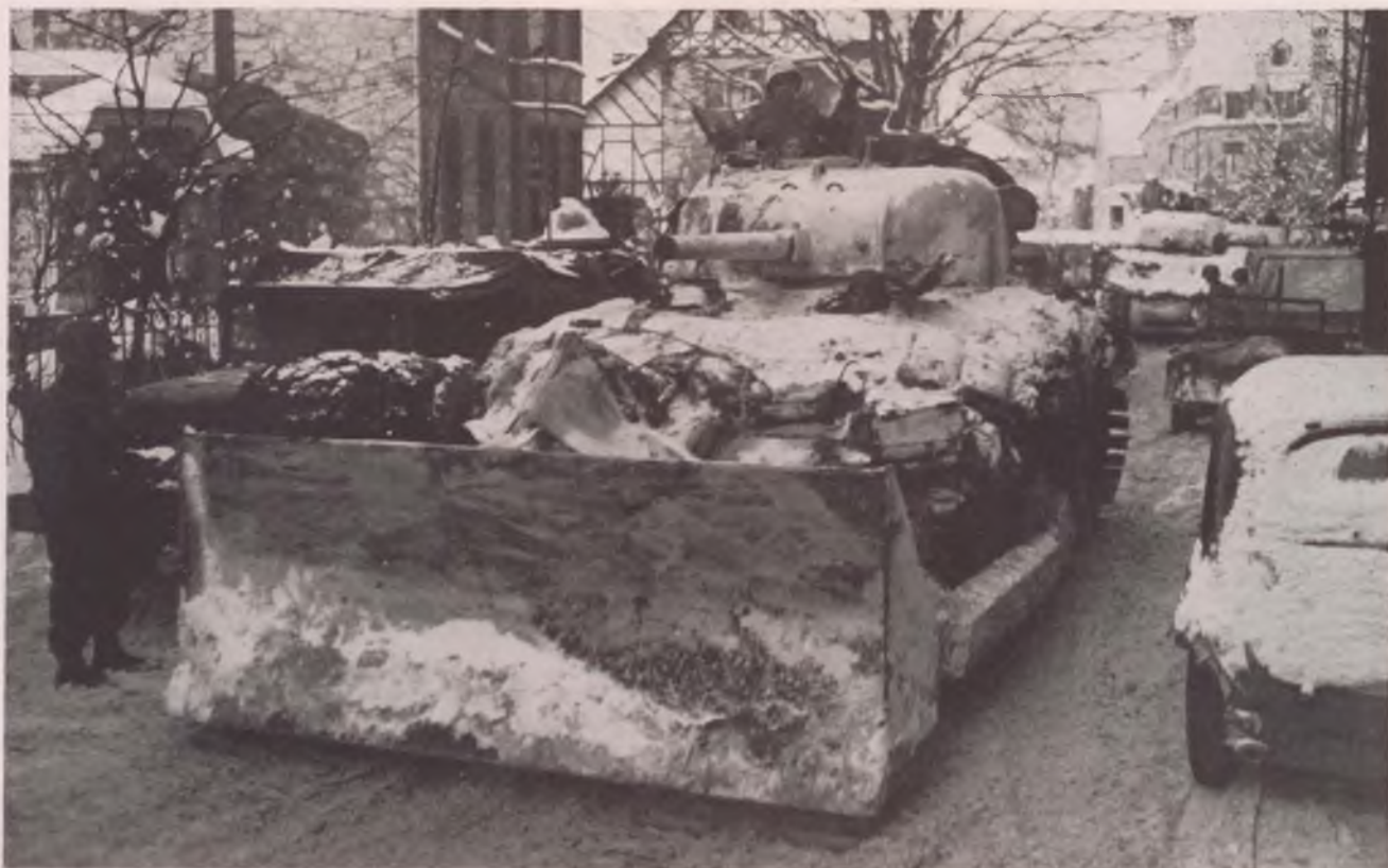
We sure needed the tankdozers
